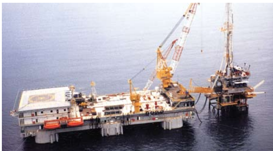
Including West Pelaut, Keppel FELS has built six KFELS SSDT™ rigs and 10 jackups for Seadrill, with another SSDT currently under construction
